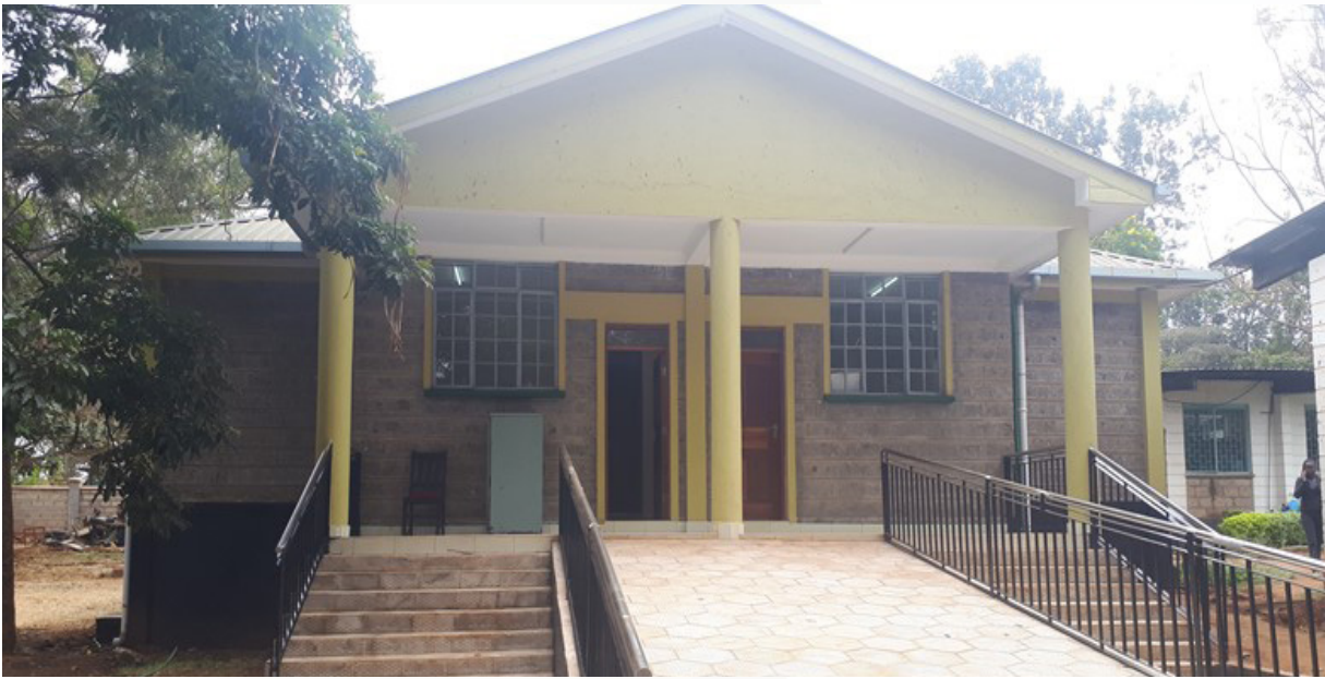
Completed ELC Twin Court in Machakos Law Courts
