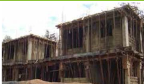
On-going rehabilitation works at Nyamira Law Court.
