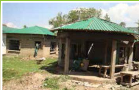
On-going rehabilitation works at Tamu Law Court.
