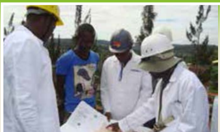
Architects discussing building design details at the Nyamira Law Court.
