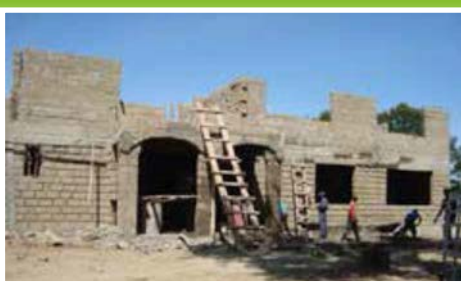
On-going rehabilitation works at Nyando Law Court.
