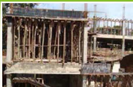
On-going rehabilitation works at Chuka Law Court.
