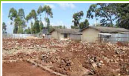
On-going rehabilitation works at Vihiga Law Court.
