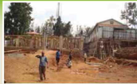
On-going rehabilitation works at Oyugis Law Court.
