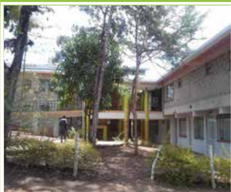
Completed rehabilitation works of Kitui and Kangema Law Courts.
