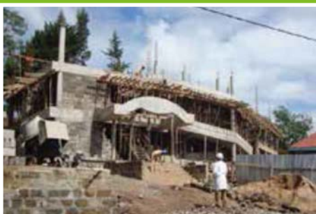
On-going rehabilitation works at Kigumo Law Court.
