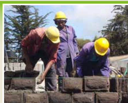
Female workers (center) are involved in the construction works.
