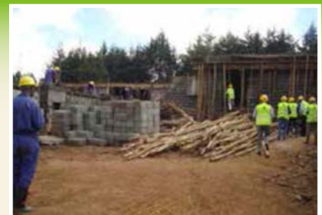
On-going rehabilitation works at Molo Law Court.
