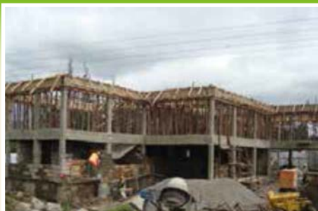
On-going rehabilitation works at Engineer Law Court.
