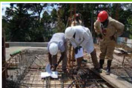
Construction Consultant supervising the construction at Kigumo Court.
