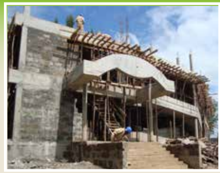
Rehabilitation works of Nine Judiciary Courts.
