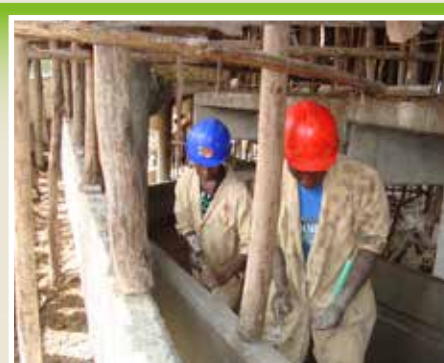
Construction workers wearing safety gears.
