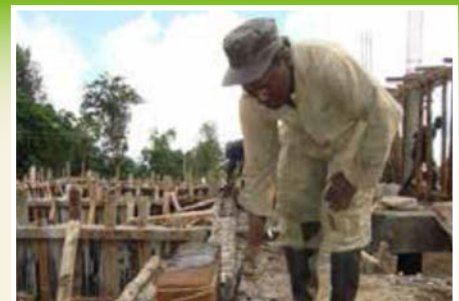
Masonry works being done at Chuka Law Court.
