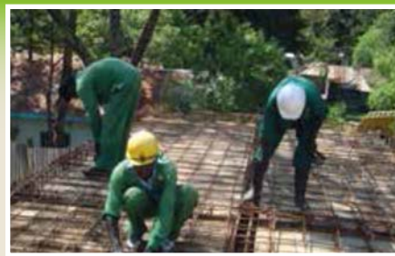
Steel works at Nyando Law Court.
